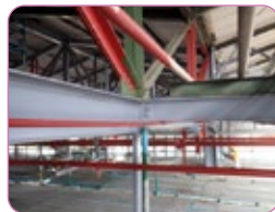
Painting of steel structures at the filling station
