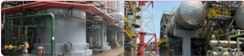
Beautification of steel structures and equipment foundations within the plant
